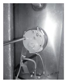
5 Unscrew the electric heater from the tank and remove it.
