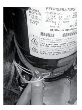
7 Remove the suction pipe and the discharge pipe from the compressor. Isolate the wires and electrical components to protect them from the burner flame when brazing the connection pipes.
