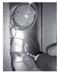
6 Remove the thermistor by hand and remove the wire sensor from the tank.
