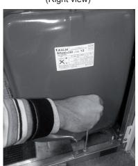
4 Unscrew the expansion vessel as shown in the picture. If the indoor unit right cover is not removed, remove the screws with a little spanner or a torque wrench.
